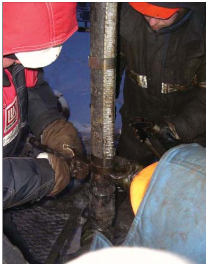
Additional equipment in the photo at left includes a wellhead system for running the cable in the well (Fig. 2; photo from Nefteservis-NN). Operators in the photo above can place the cable inside or outside of the tubing, as shown here (Fig. 3; photo from Nefteservis-NN).
