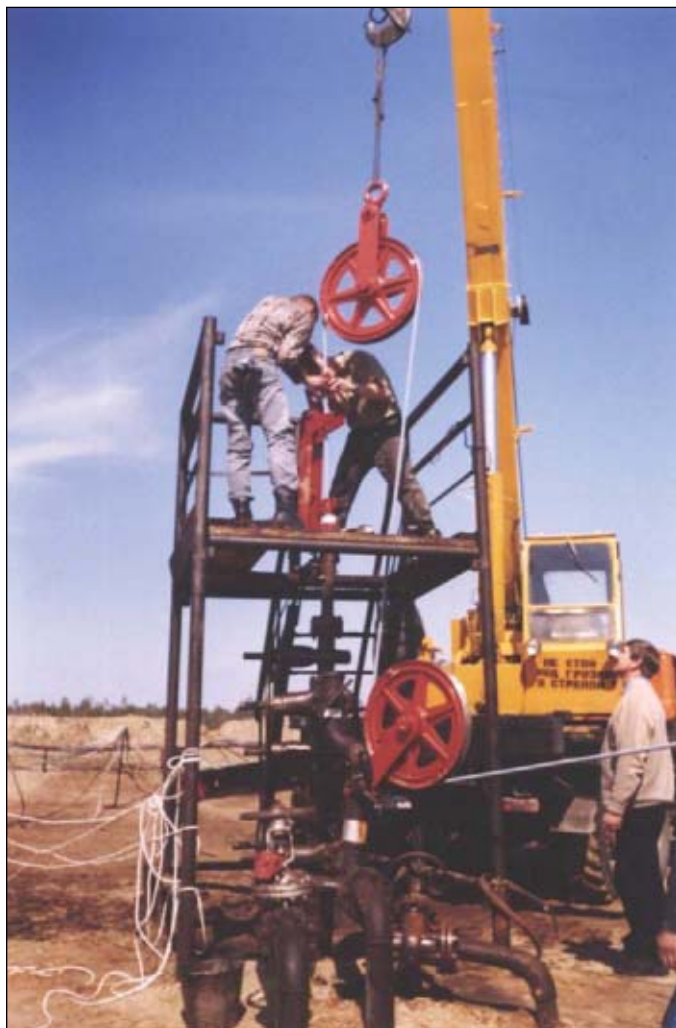
Additional equipment in the photo at left includes a wellhead system for running the cable in the well (Fig. 2; photo from Nefteservis-NN). Operators in the photo above can place the cable inside or outside of the tubing, as shown here (Fig. 3; photo from Nefteservis-NN).
